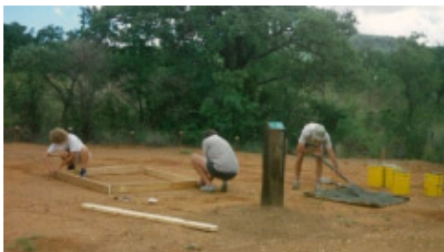
First slab -start
